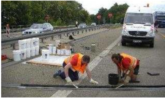
Figure 8. Application of primer to substructure
