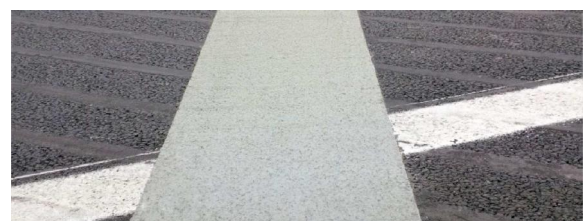
Figure 1. A Polyflex®Advanced expansion joint
