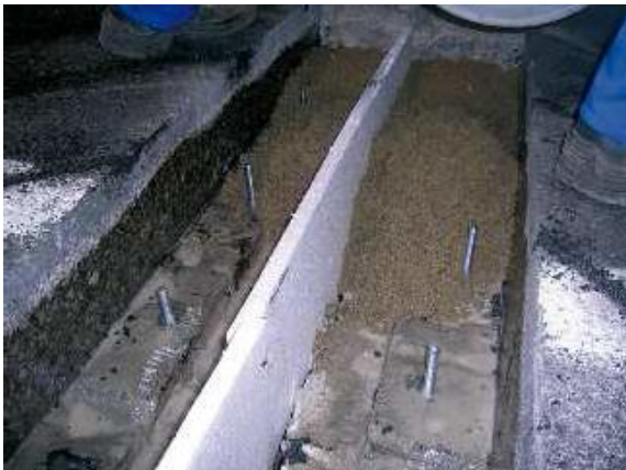
Figure 9. Forming polymer concrete base
