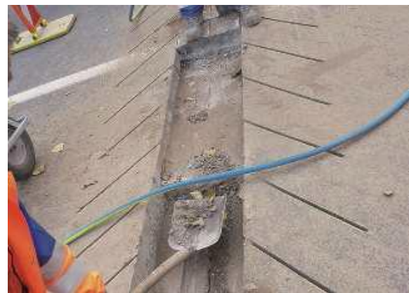
Figure 6. Removal of old joint/surfacing as needed
