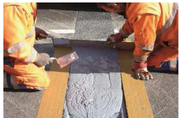
Figure 13. Precise levelling of material to road surface
