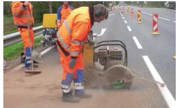
Figure 5. Cutting of surfacing across the joint
