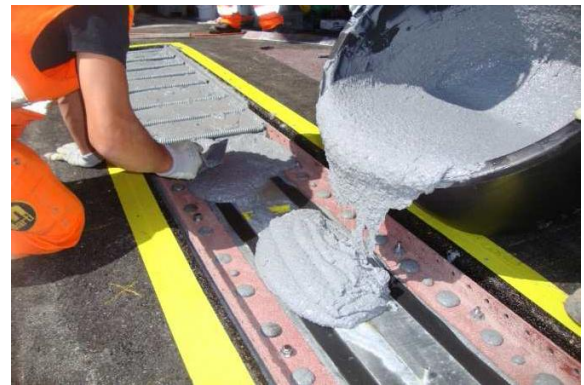
Figure 12. Placing of PU material
