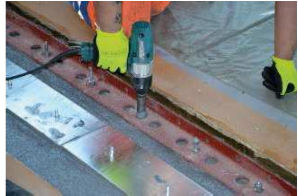
Figure 11. Fixing of angles, and plate across gap
