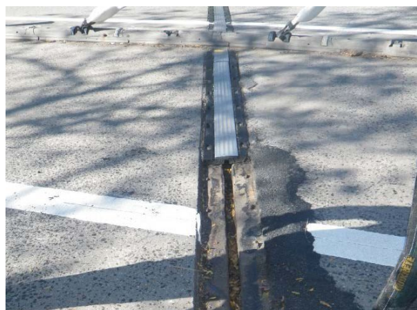
Figure 18. Existing expansion joint after removal of one particularly deteriorated section
