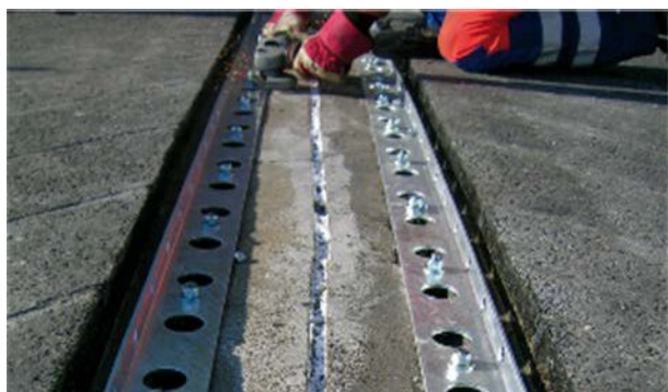
Figure 8. Fixing angles to polymer concrete base
