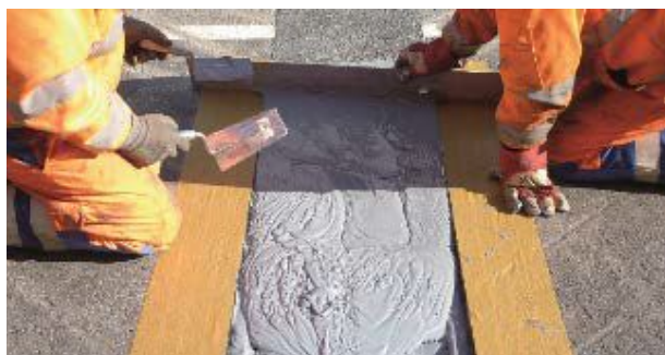
Figure 9. Precise levelling of material to road surface
