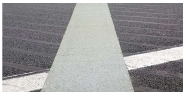
Figure 1. A Polyflex® Advanced plug expansion joint
