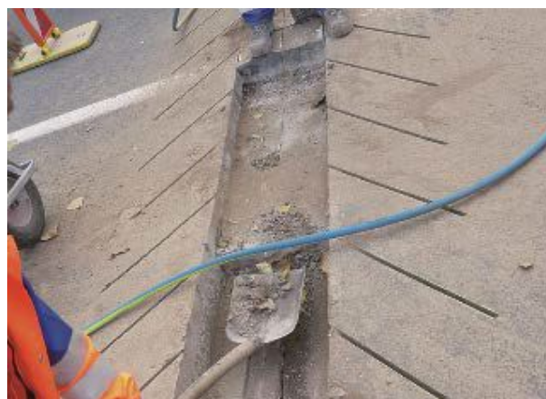
Figure 5. Removal of old joint/surfacing as needed
