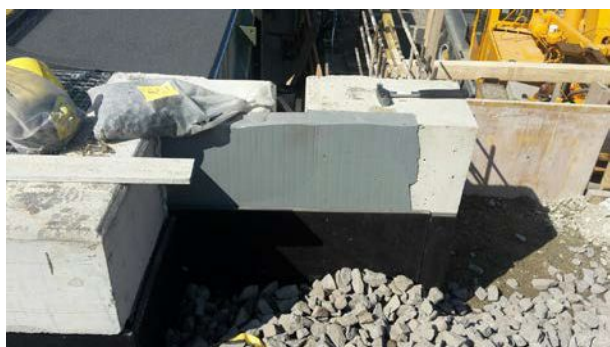
Figure 17. Upstand at end of railway joint following removal of formwork and placing of protection mat (black) and track ballast (stones)
