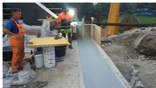
Figure 16. Polyflex®Advanced joint as placed, showing formwork for upstand at one end
