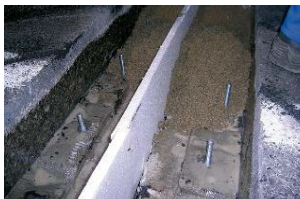
Figure 7. Forming polymer concrete base
