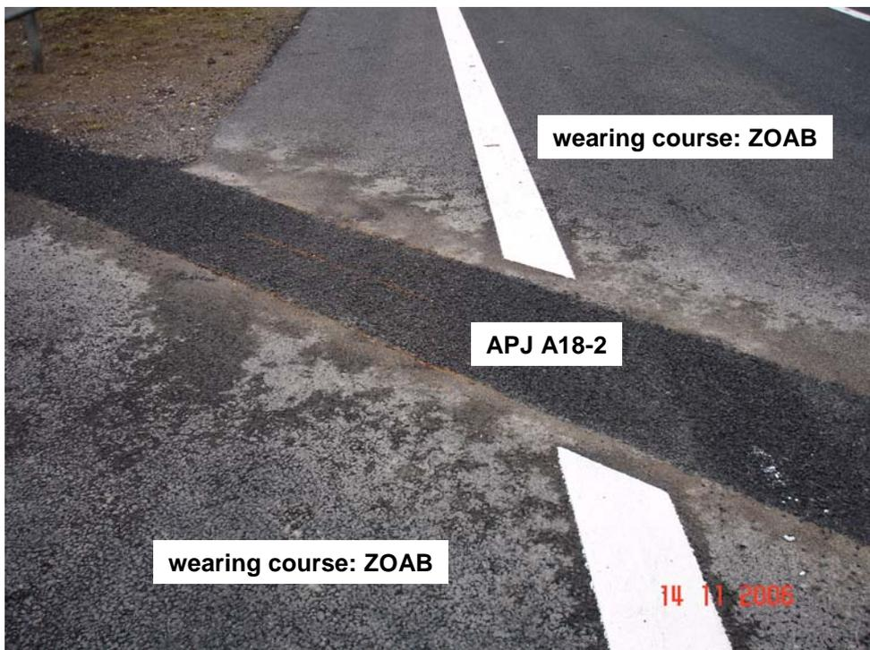
Figure 6.3.2: Appearance of surface dressing of the APJ A18-2
