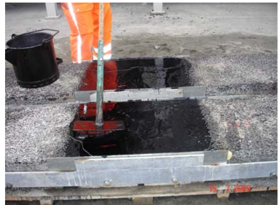
Figure 5.1.18: Application of the surface dressing without the use of small sized aggregates
