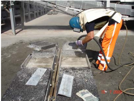
Figure 5.1.7: Sand blasting the surface of the concrete slabs and of the vertical surface of the bridge pavement
