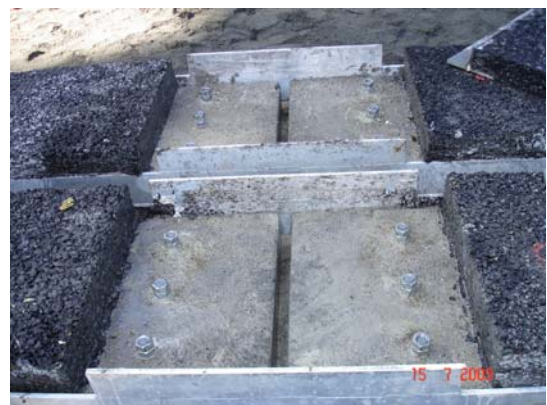
Figure 5.1.6: After fixing, the anchor rods were let cure during the curing time of approx. 30 min
