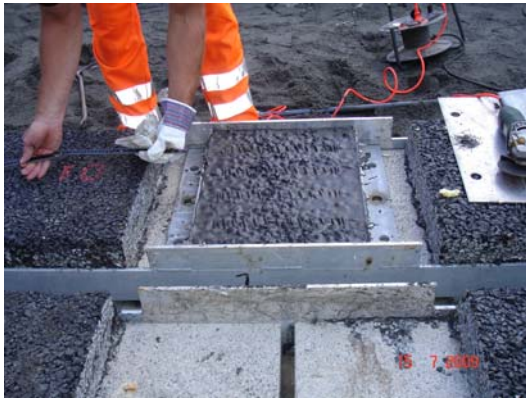
Figure 5.1.3: Placement of the joint module onto the middle of the joint gab
