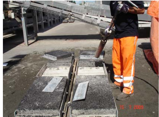
Figure 5.1.8: Activation of the adjoining surface of the pavement using hot air
