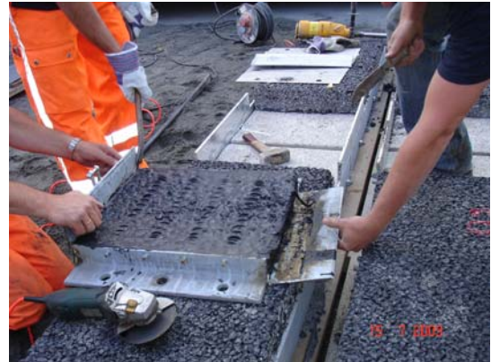
Figure 5.1.2: Removing the metal barrier plate from the prefab joint module
