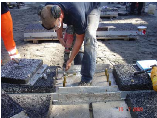
Figure 5.1.5: After inserting the capsule (with chemical resin) into the holes, the metal anchor rods were installed with a rotary hammer
