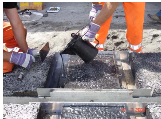
Figure 5.1.12: Pouring the hot binder into the gap between the joint module and the bridge pavement
