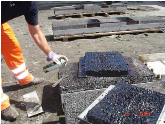
Figure 5.1.9: Priming the T-metal profile of the prefab joint module
