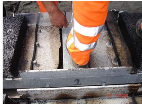
Figure 5.1.10: After stuffing the foam caulking, hot binder was poured onto the surface of the concrete slab, and then a metal bridging plate was placed
