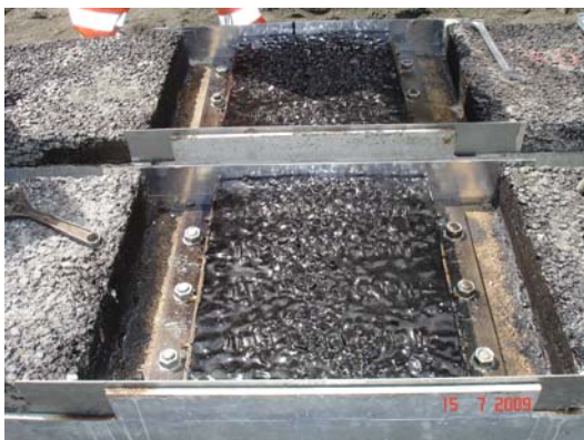
Figure 5.1.11: The prefab joint modules were fixed onto the concrete slabs
