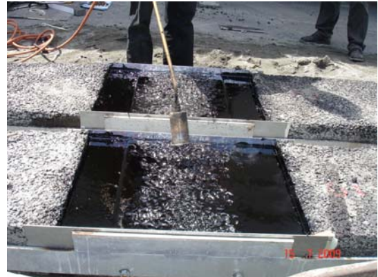
Figure 5.1.14: Heating the surface of the prefab module with a gas-flame
