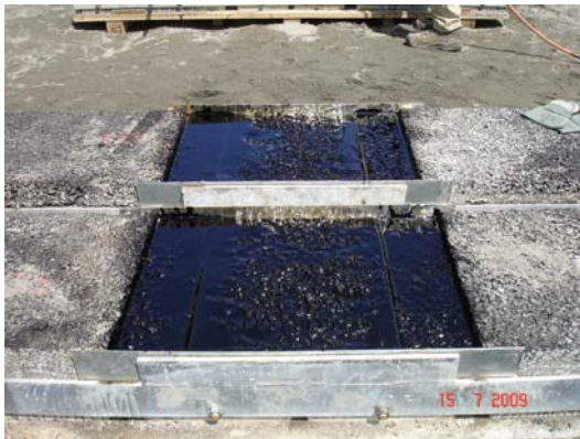
Figure 5.1.15: After pouring the hot binder on the surface of the prefab module and both new build joint stripes
