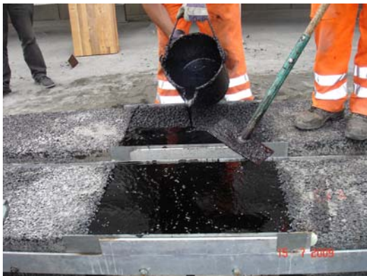
Figure 5.1.17: Pouring the hot binder onto the compacted aggregates
