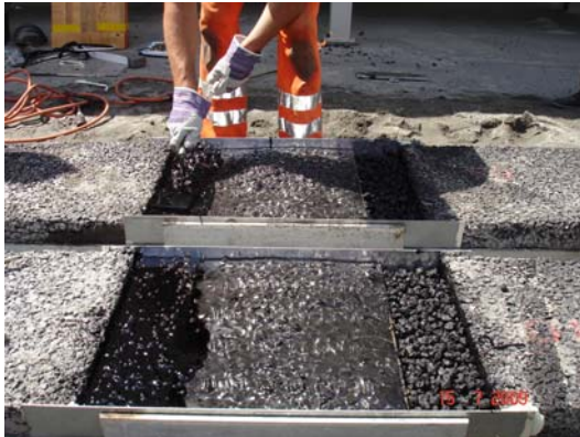
Figure 5.1.13: Application of both joint stripes between the joint module and the bridge pavement
