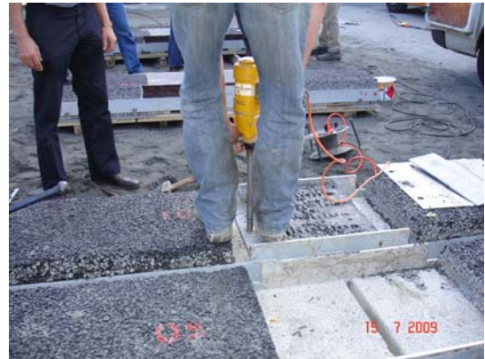
Figure 5.1.4: Drilling anchor holes with rotary hammer to fix the joint module onto the concrete slabs using chemical anchor
