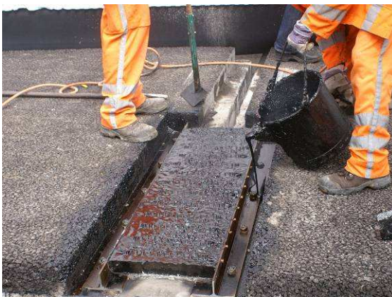
Application of bituminous binder after tightening of the bolts that anchor the prefab element.
