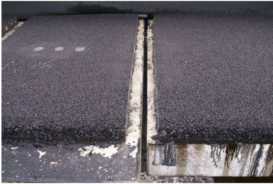
Left: Situation at start of prefab element installation. Right: Cutting of joint trough.
