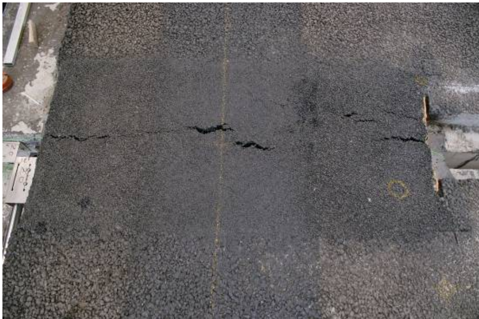
Figure 30. Impression of the -13 mm joint after failure.
