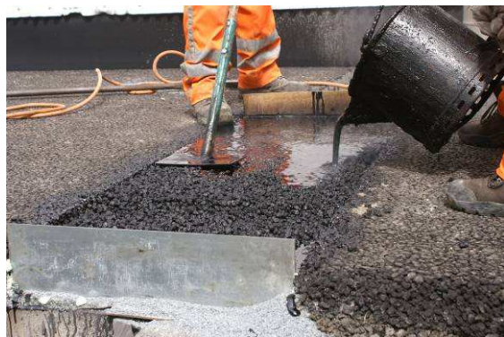
Filling of the trough with prefab joint element. Left: Levelling of the skeleton of pre heated mineral. Right: Bituminous binder is worked into the skeleton of pre heated mineral.
