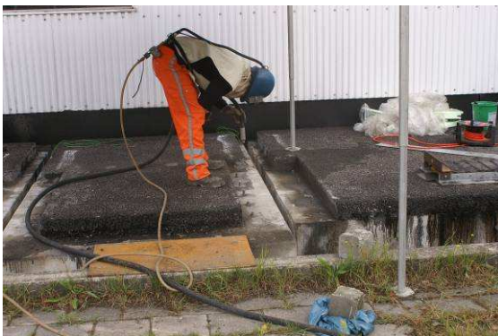
Left: Sandblasting of concrete substrate. Right: Heating of adjacent asphalt structure.
