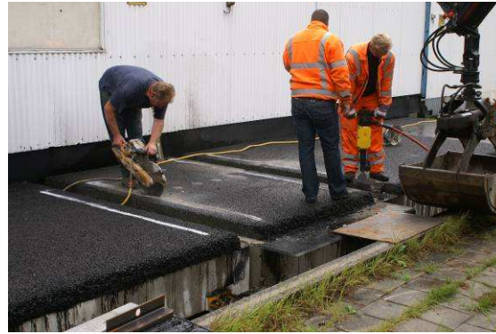
Left: Situation at start of prefab element installation. Right: Cutting of joint trough.
