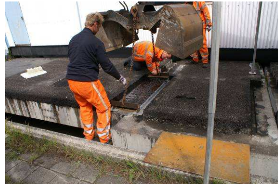
Left: Installation of joint bridging strip. Right: Installation of Prefab Silent Joint.
