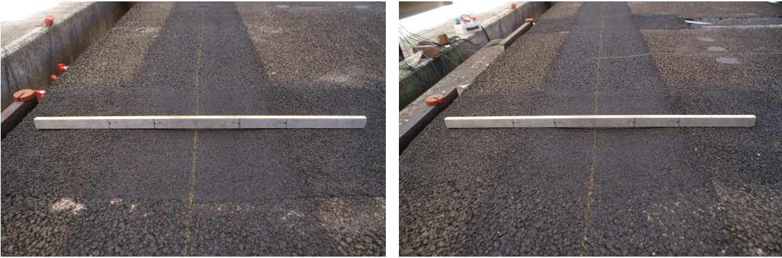
Rutting at N=85000. Left: +13 mm joint, right: -13mm joint.
