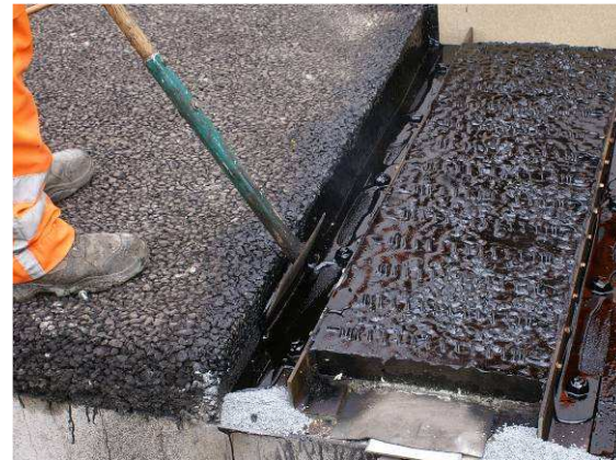
Application of bituminous binder after tightening of the bolts that anchor the prefab element.
