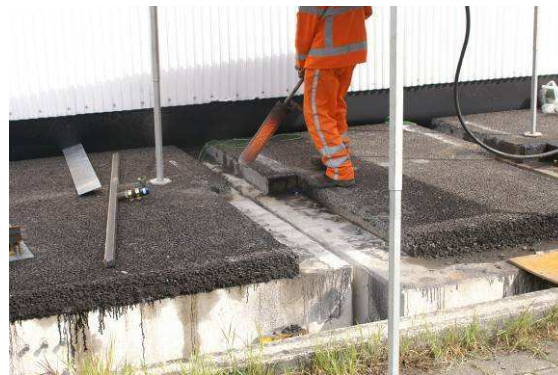
Left: Sandblasting of concrete substrate. Right: Heating of adjacent asphalt structure.
