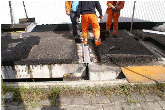
Left: Installation of joint bridging strip. Right: Installation of Prefab Silent Joint.
