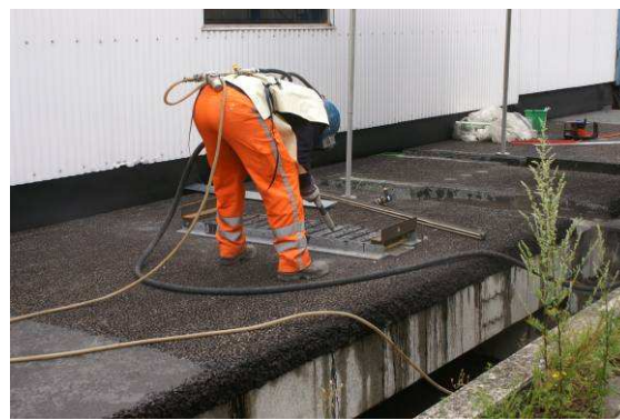
Left: Joint substrate repair. Right: Sandblasting of prefab Silent Joint.
