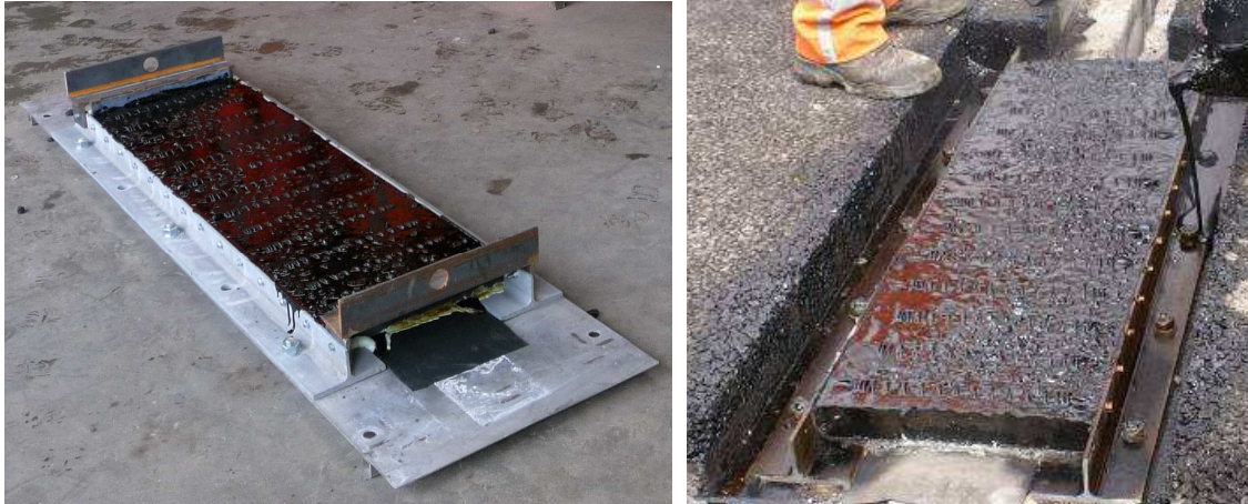
Figure 1. Left: Prefab Silent Joint element at contractors yard. Right: prefabricated element anchored to concrete substrate at LINTYRACK site.
