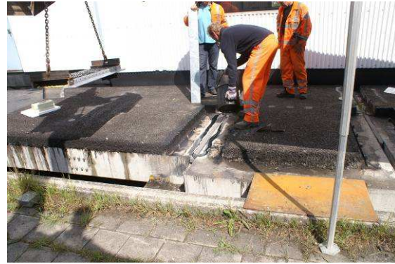
Left: Application of compressive bedding. Right: Installation of bituminous material for embedment of metal strip.
