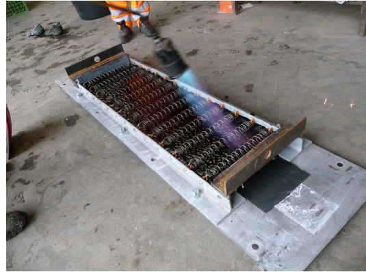
Construction of prefab element at contractor's yard. Left: Installation of springs after application of lower bituminous layer. Right: heating of springs and lower joint body layer.
