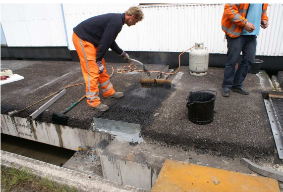
Application of small sized chippings on the Prefab Silent Joint surface.
