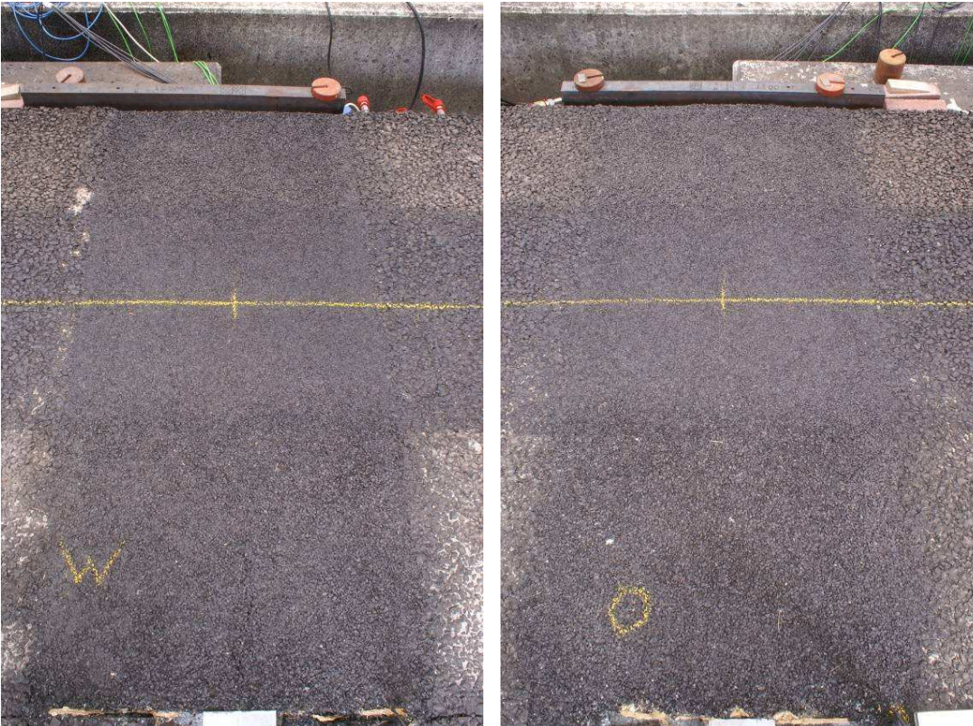
Top view at N=70000. Left: +13mm joint, right: -13mm joint.
