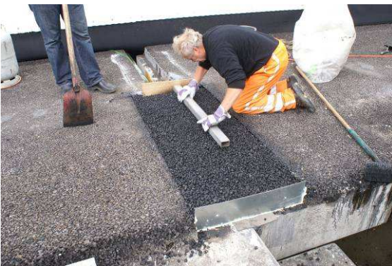
Filling of the trough with prefab joint element. Left: Levelling of the skeleton of pre heated mineral. Right: Bituminous binder is worked into the skeleton of pre heated mineral.
