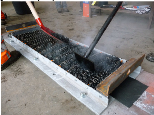
Construction of prefab element at contractor's yard. Left: application of pre heated mineral for second joint body layer. Right: application of binder into second layer.
