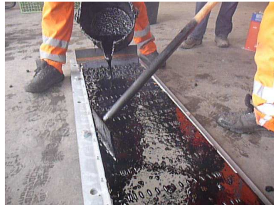
Construction of prefab element at contractor's yard. Left: application of pre heated mineral for second joint body layer. Right: application of binder into second layer.
