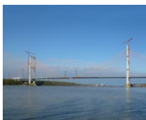
Audubon Bridge (USA)
