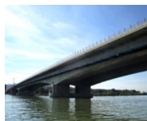
Traismauer Bridge (AT)
