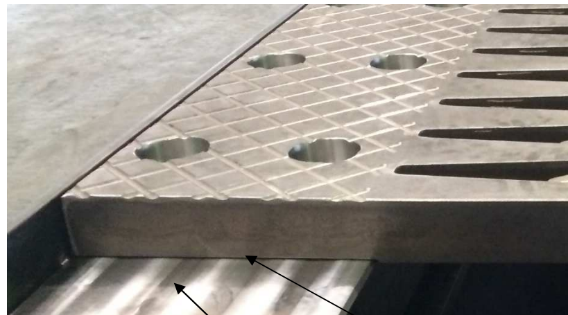
mechanically processed substructure and finger plates!
